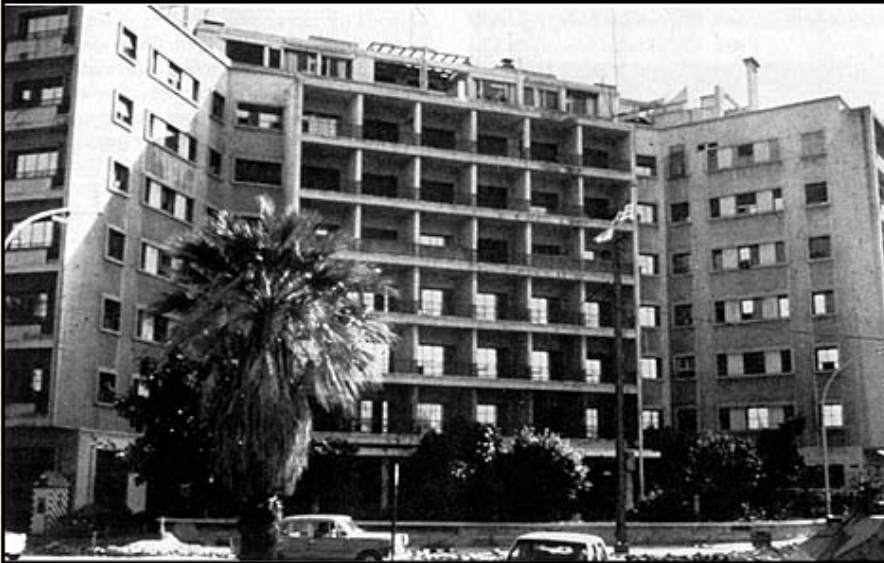
The American Embassy in west Beirut, as it appeared before the April 18, 1983 bombing.
