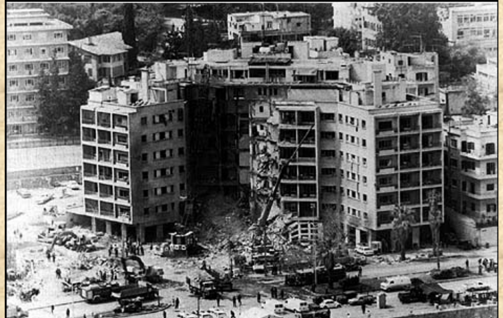
An aerial view of the American Embassy as heavy cranes continue to remove rubble from the upper floors on 21 April, 1983, following the terrorist bombing three days earlier.
