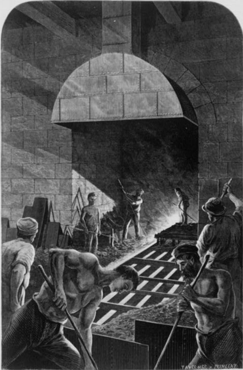
THE MANUFACTURE OF IRON.—TAPPING THE TUNDRAC.—(Taken at Tipton, and Printed.—(See Page 964.)
