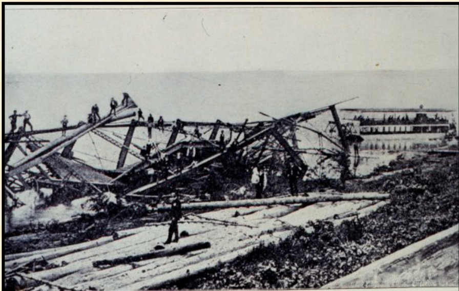
RUIN CAUSED BY THE FLOOD
